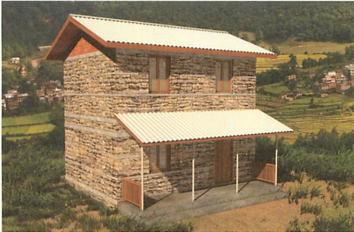
Figure 5.2 An Earthquake-Resistant Model House
